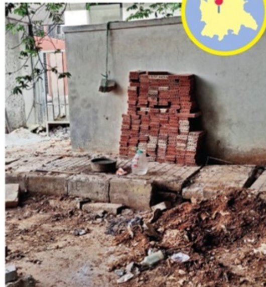
The footpath outside Godrej Woodsman on the Dasarahalli Road needs attention.
