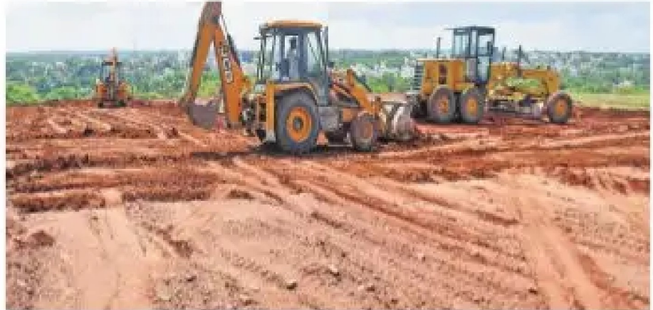
Earth movers at work on vacant land at Visvesvaraya Layout near Kengeri to prepare a makeshift helipad for PM Narendra Modi, on Thursday | VINOD KUMAR
