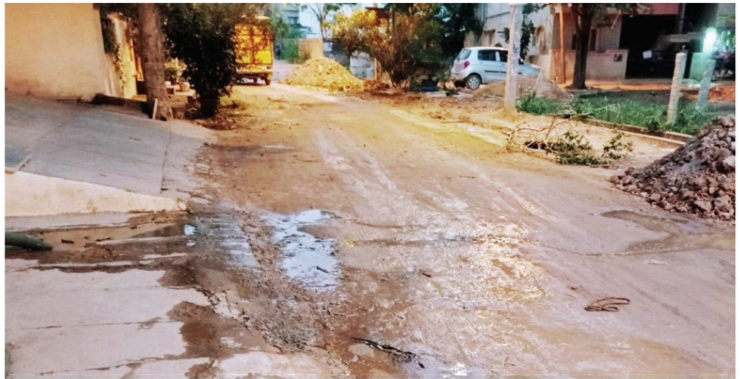
Sewage overflows to the main road from a soak pit dug by a high-rise building owner at Meenakshi Layout
