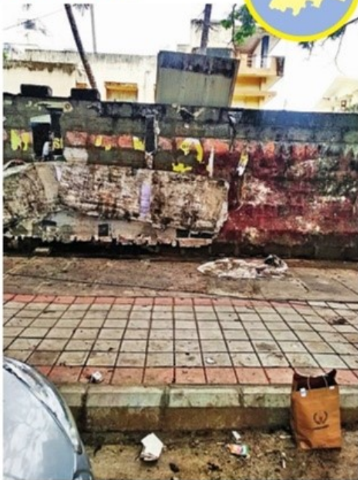
Jayanagar 9th main road, 5th block was well maintained earlier. Film posters put up by cinema halls have made the walls dirty and dull. BBMP should ban this.
