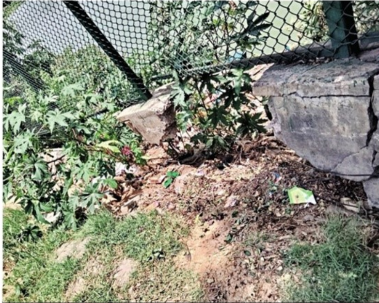
Condition of retaining wall of Hebbal lake
